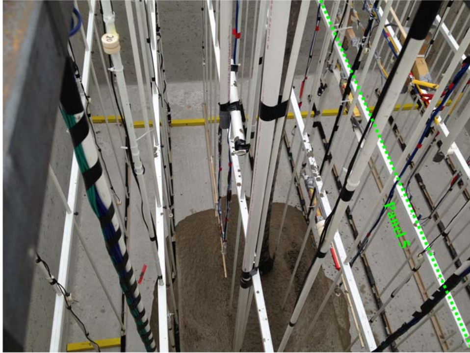
Figure 5.6 Concrete pouring into the concrete test cube after panels were deployed.
